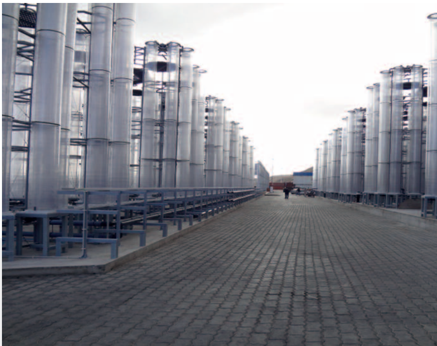
Figure 4: BFS's Demonstration Plant, near Alicante
